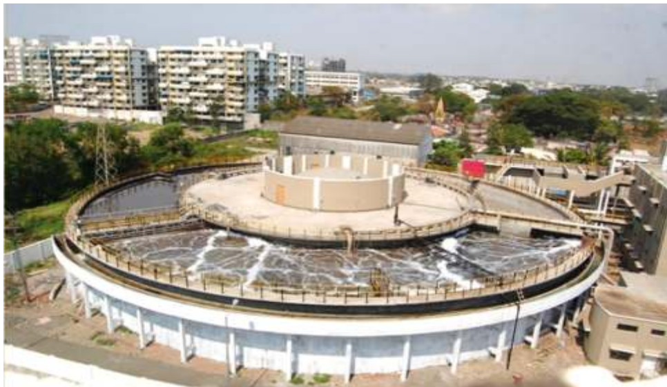
30 MLD SEWAGE TREATMENT PLANT AT AKURDI ON COMBITREAT TECHNOLOGY
