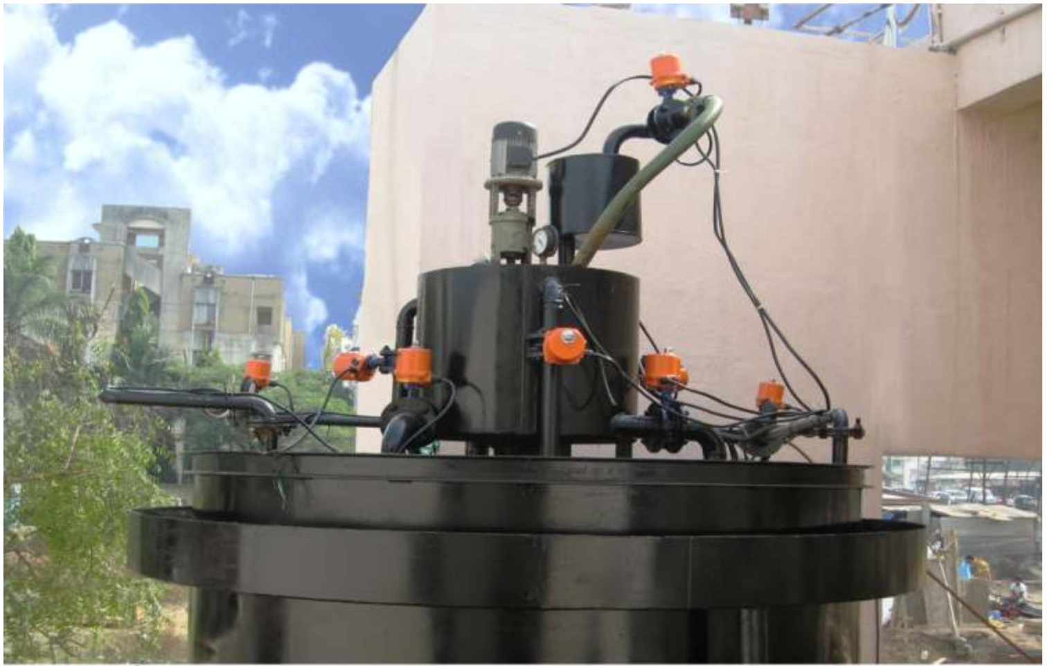
180 M 3 / DAY CAPACITY PACKAGE SEWAGE TREATMENT PLANT AT NANDED.
